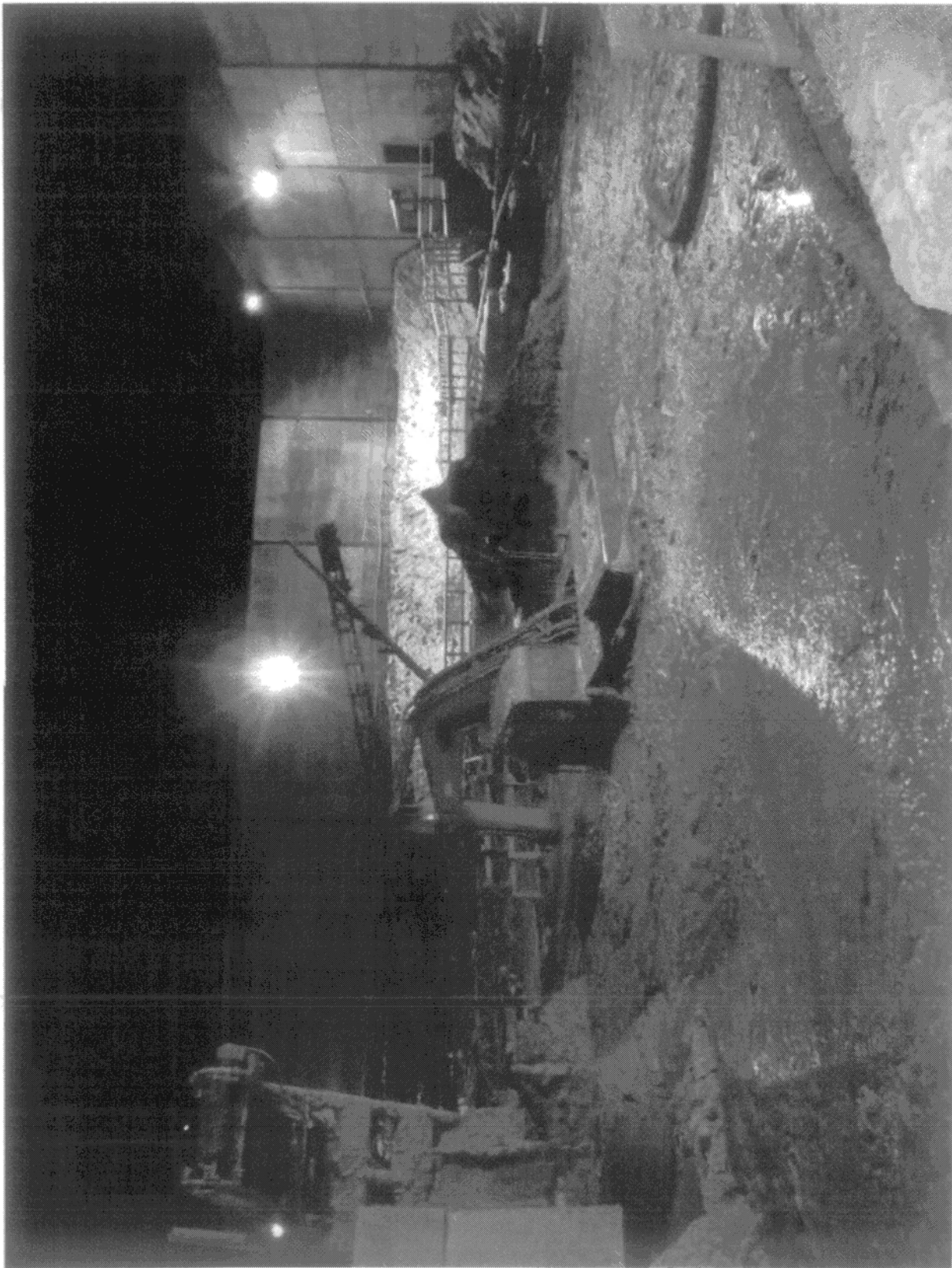
Central North Kenmore Portal (P44) Equipment 2008-12-16 06:59:30 J:\Photographs\Central\2008\12 - December 2008\BWC-06993.jpg Roger Johnson North Kenmore Portal - 12-16-08 - A Hatachi 330 excavator
